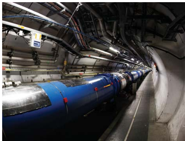
Fig 1. LHC accelerator tunnel , 2014, Chris Henschke, photograph. Image courtesy of the author.
