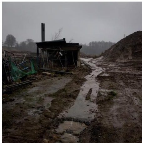
Figure 71 (Plate #37) - Site previously occupied by the Star Paper Mill (opened in 1875), being prepared for five hundred new homes at Feniscowles, Blackburn. Harrison, December 2018
