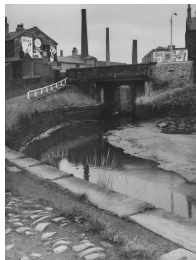
Figure 13 - Draining of the Locks, 1957, Elizabeth Ashworth, www.CottonTown.org archive, accessed 3 August 2018
