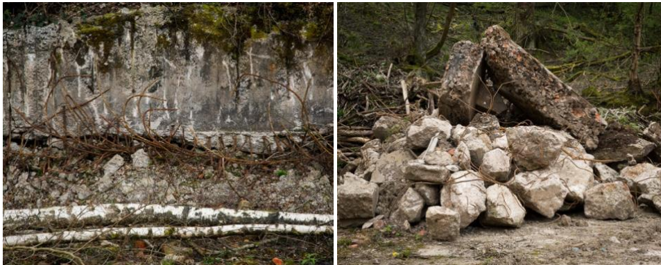
Figure 74 (Plate #42) – Fragments of building material from the former Star Paper Mill, being broken up to form the foundations for a new suburban housing development along the banks of the River Roddlesworth. Harrison, 2019.
