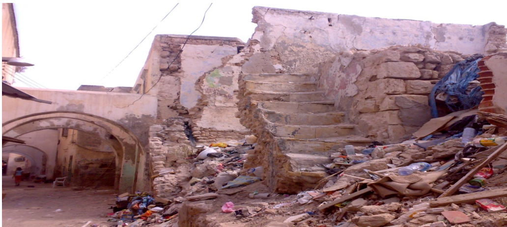
Figure 7.16: The damaged old and new houses in the old city of Tripoli..
