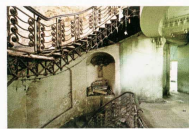
Tiring Department Store, Cairo, 2010 Designed by Oscar Horowitz for Les Grands Magasins, the Tiring Department Store opened its doors in 1912. The luxurious store matched the elegance of similar establishments in Paris, such as Galeries Lafayette. After the revolution of 1952 the Egyptian government nationalised it.
