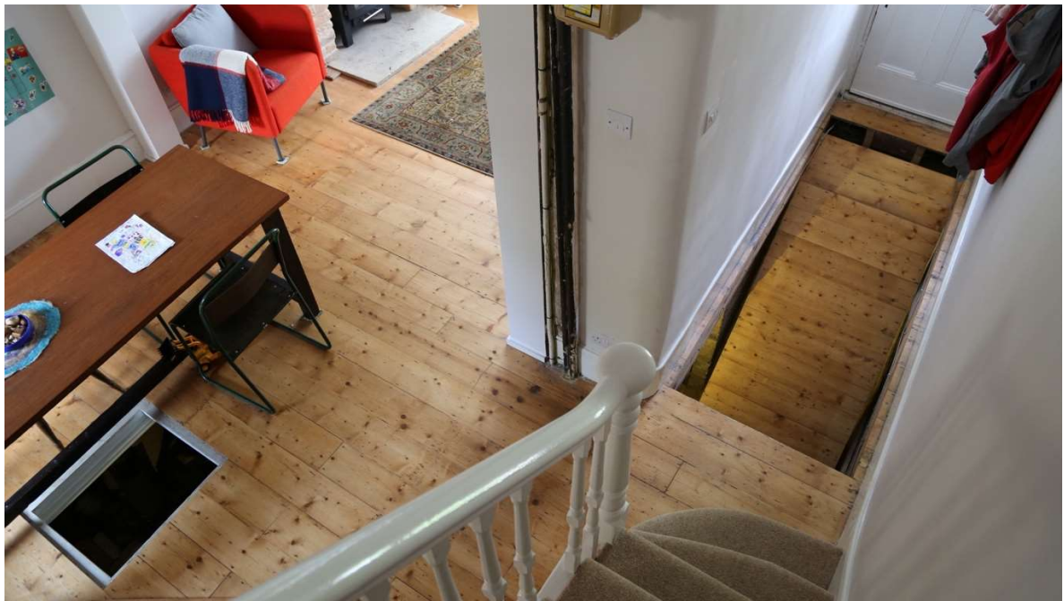
Figure 114; 22 St John Terrace, trap door and hallway ramp, London, Theo Harper, 2013-2016.
