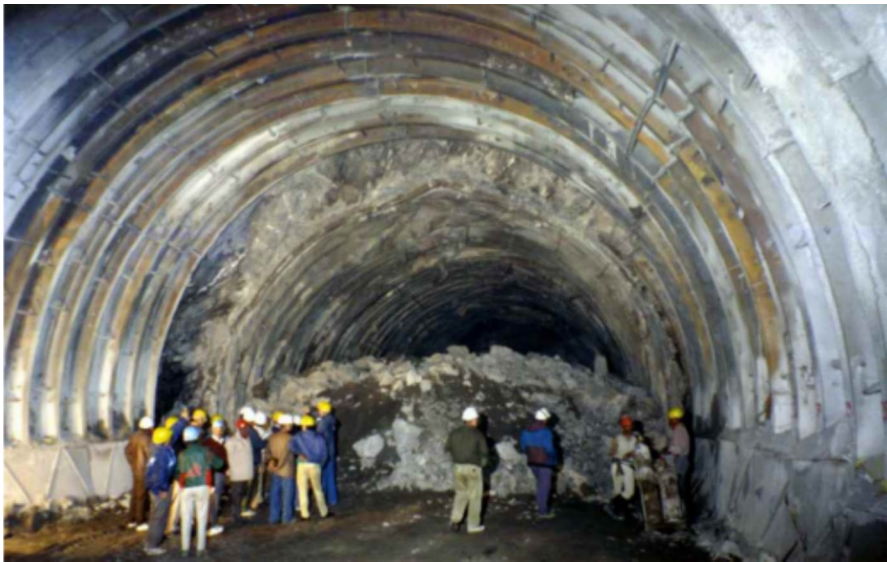
Fig. 1 Typical squeezing failures from field case study (Hoek. 2001)
