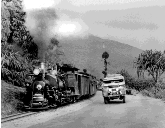
Figure 7: 1: Photo Courtesy David Charlesworth
